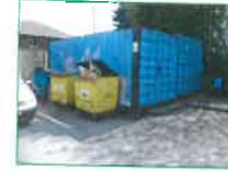
CONTAINERS 2 & 3 : 6 m x 2.4 m x 2.6m high
